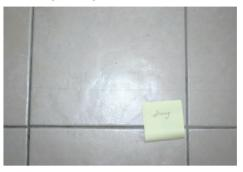
Figure A4.3: Cracking of ceramic floor tiles over a shrinkage control joint in a floor not affected by earthquake
